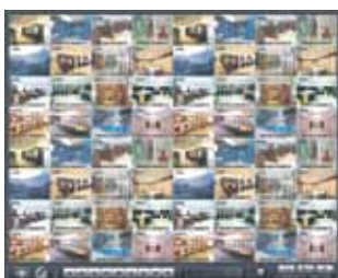
Central Monitoring System (CMS)
